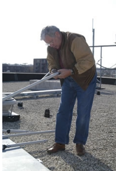
Larry, W9OKI , hard at work on the roof.
